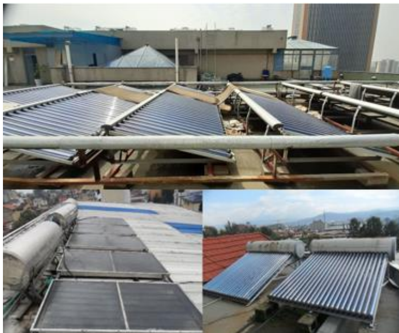
Figure 4-10: Some of the SWHs systems in hospital and health specialty centers
