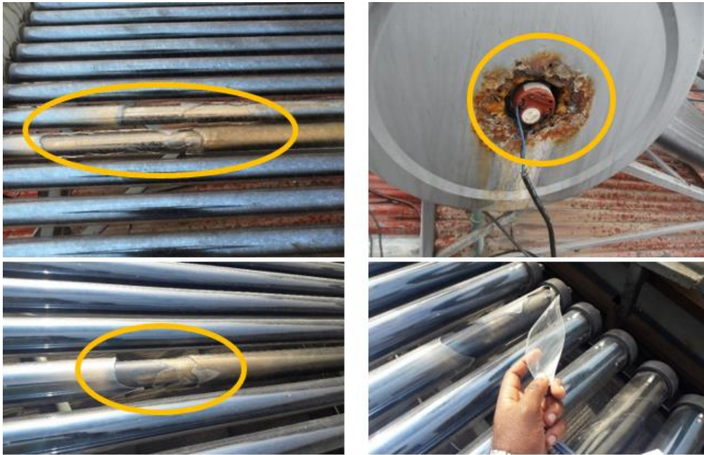
Figure 4-22: Evacuated tube collector type SWH under poor working condition
